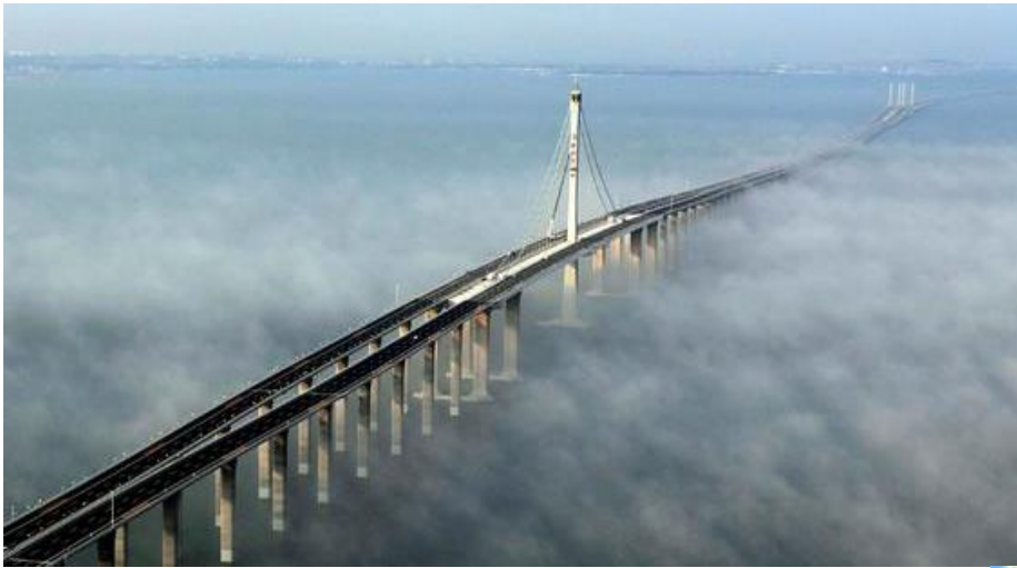
Jiaozhou Bay Bridge
